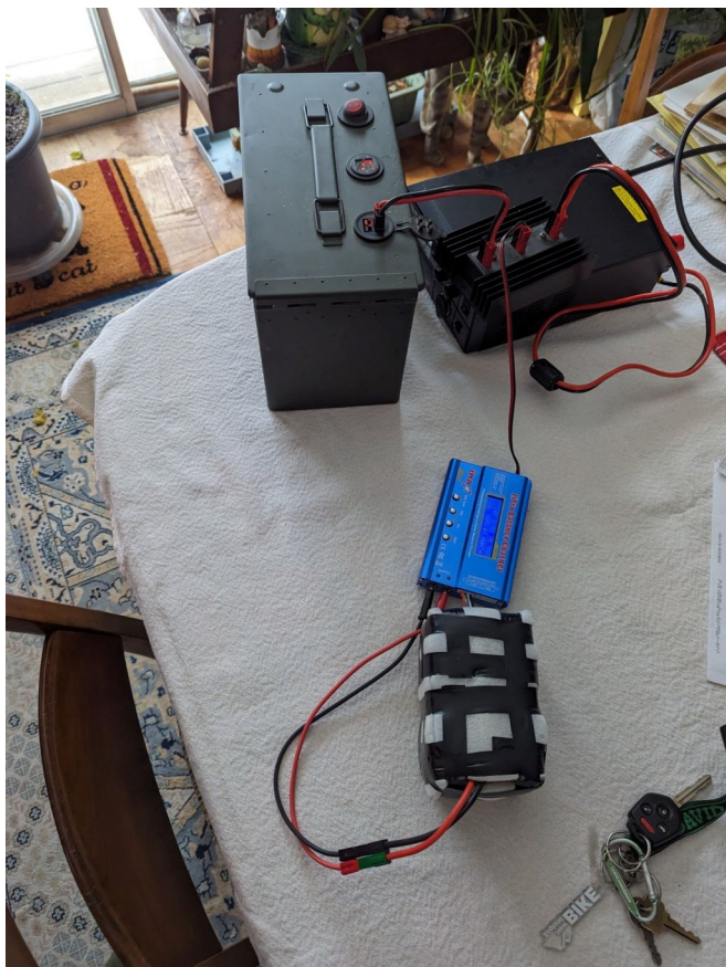
Charging the Batteries
